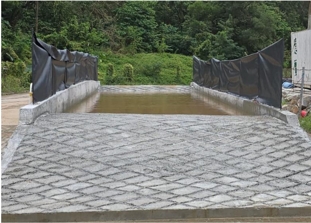
Photo 5 – Additional wheel washing facility provided on site.
